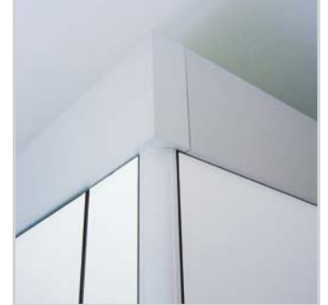
PRIMO F/K: Corner design for carriers for suspended system
