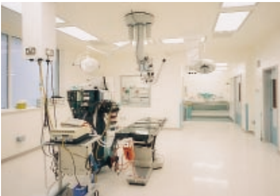
Top - MAT Technologies, UK Bottom - Northampton General Hospital, UK
